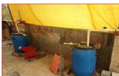
Plate5.1: Digestion Tank with Air Pillows
